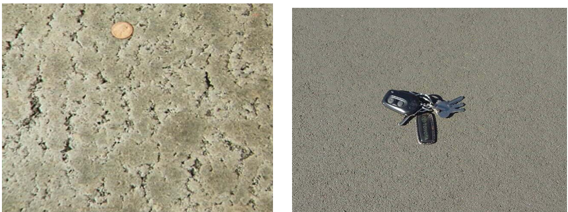
Figure 1 – Examples of RCC Pavement Surface Finish
