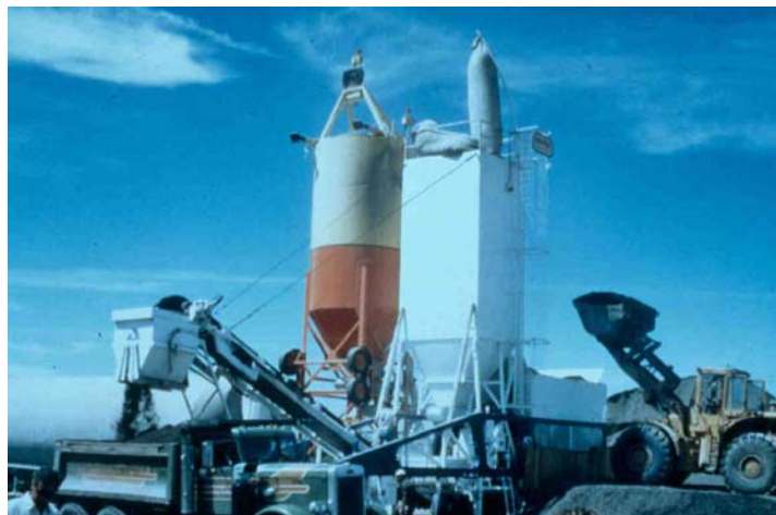
Figure 5 – A Pugmill Plant with a Gob Hopper
