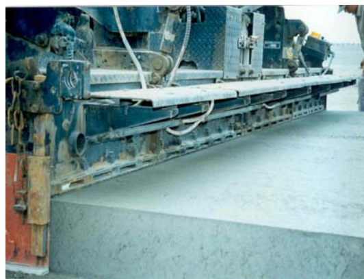
Figure 2 – Extruded RCC from a High Density Asphalt Paver
