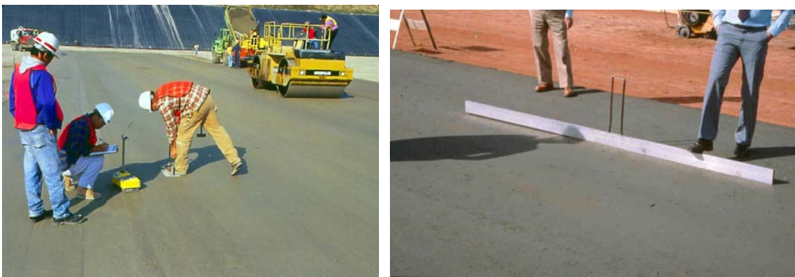
Figure 7 – Density and Smoothness Testing
